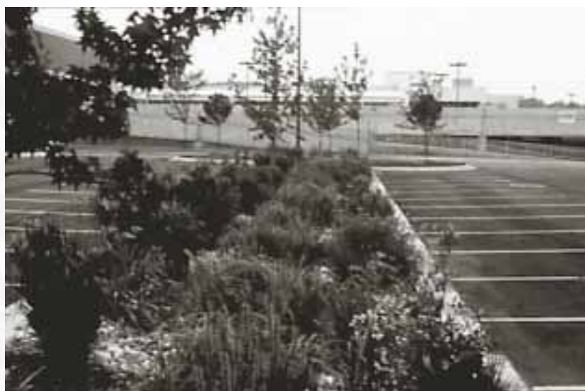
Figure 1-1. Parking lot bioretention area
